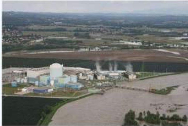
Krško Nuclear Power Plant
